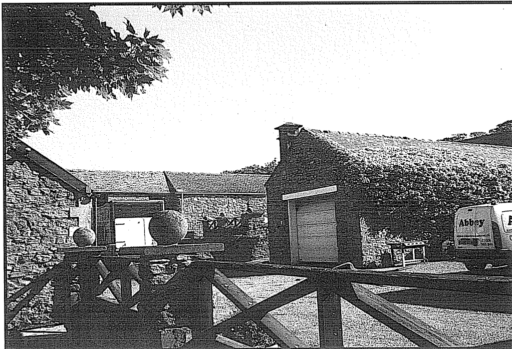
A3.4 : View North to Sunniside farm stable yard
