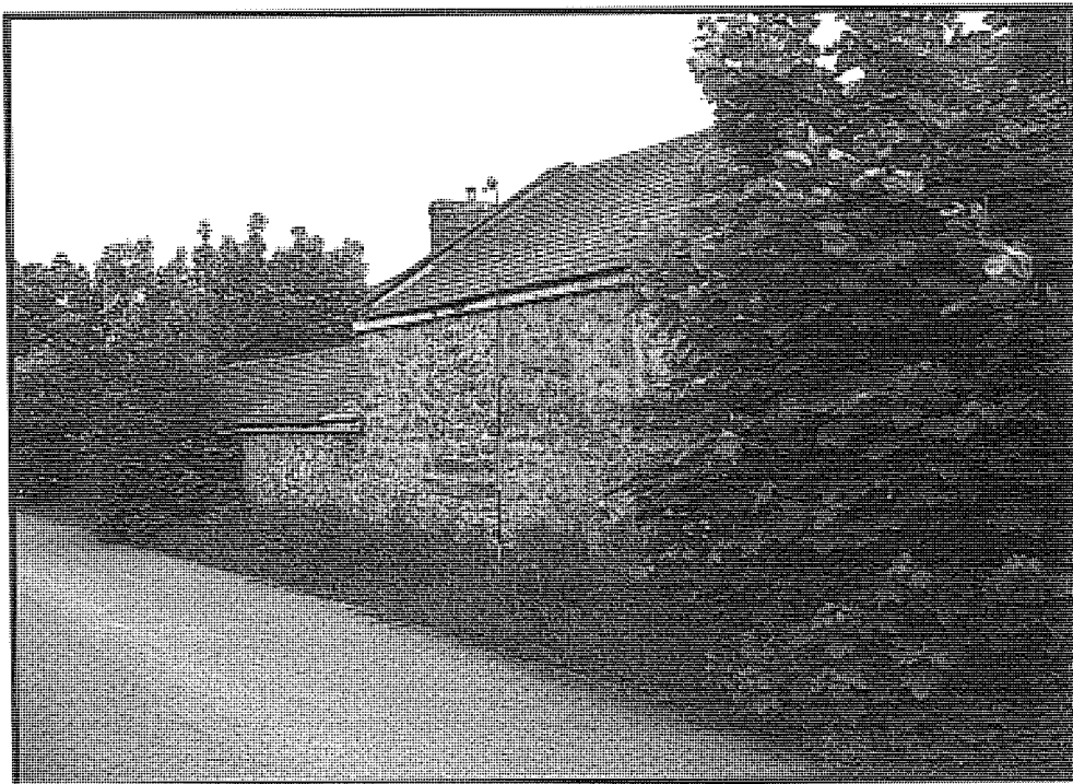
A3.6 : View SSW of east elevation of east range of farm (Scale 3m)
