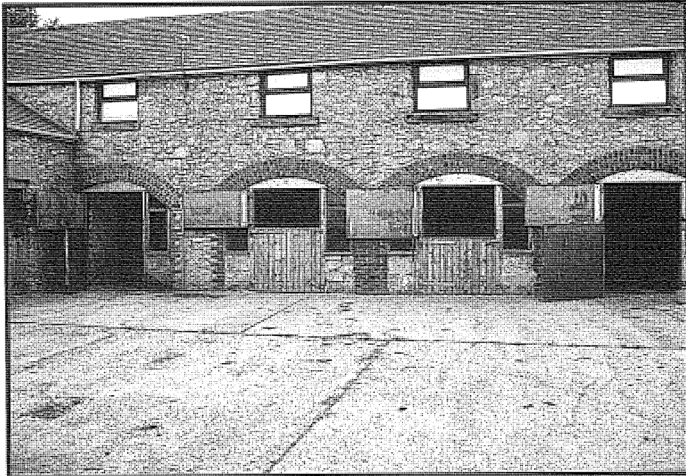
A3.16 : Stable block (5) from the west, Scales 2m
